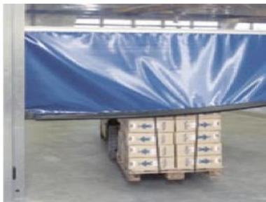
2. The Curtain can then be reset by opening the door to its top limit, allowing it to relocate back into its guides which will happen automatically.
