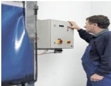
3. By pressing the lower switch the door will then close allowing the curtain to revert back to its normal state.
